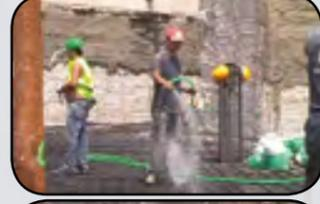
4 Place the **MAXJOINT® W-SEAL**, water-swelling profiles along the foundation perimeter using the **MAXFLEX® 100 W** polyurethane-based sealant and concrete nails each 30 or 40 cm to fix the profiles onto concrete surface. When small surface damages, use **LEAKMASTER** for filling before placing the profiles.
