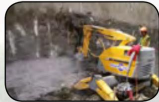
1 Prepare the substrate, and patch damages/holes on the retaining wall surface using any suitable structural repair mortar: **MAXREST®** or **MAXRITE®-F**.
