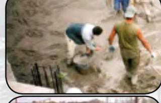
7 Apply **MAXSEAL® SUPER** by dry-shake method, providing a uniform coating on surface to be waterproofed.
