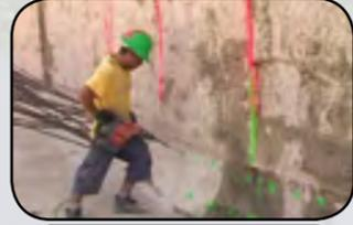
2 Apply two coats of the **MAXSEAL® SUPER** waterproofing mortar with osmotic performance.
