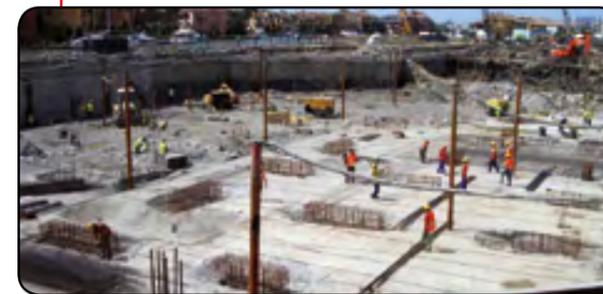
Applying **MAXSEAL® SUPER** on slab reinforcement prevents any deterioration of the waterproofing, and moreover, the proposed system can be adapted to work progress without causing delays or interference with other areas.
