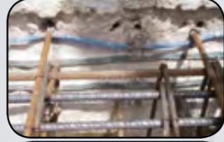
3 Insert the bars into the foundation slab-retaining wall connection area using the **MAXFIX® E** or **MAXEPOX® FIX**. Seal of areas around the bars with the **LEAKMASTER** water-swelling sealant is highly recommended.
