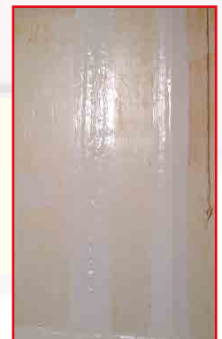
Covering of the rods with MAXEPOX® CARBOFIX .
