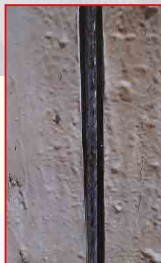
Placing of rods inside of the groove.
