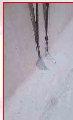
Anchoring of the rod into the slab using MAXFIX® -ER .
