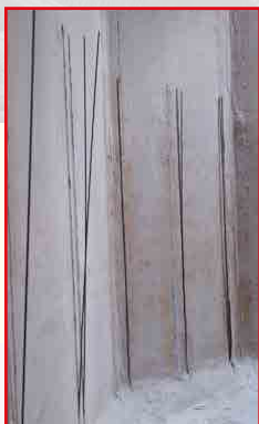
Preparation of the strengthening with DRIZORO® CARBOROD .
